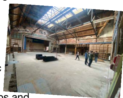
The 'old ballroom' about to be refurbished
